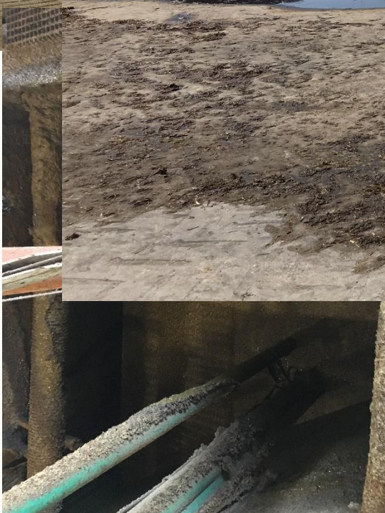
The sand-cleaned slurry is pumped through a pipe to the BMJ
